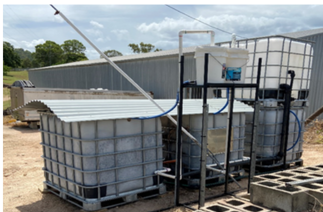
Figure 1. Koumala commercial biobed site.
