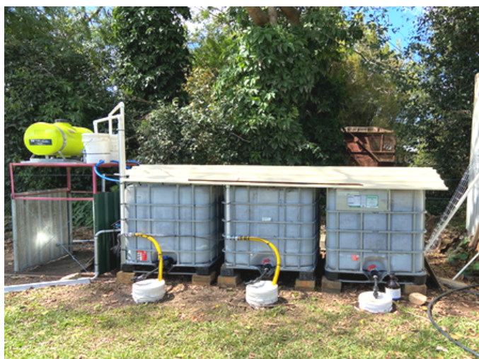
Figure 1. Biobeds at Farmacist's Sandiford office.
